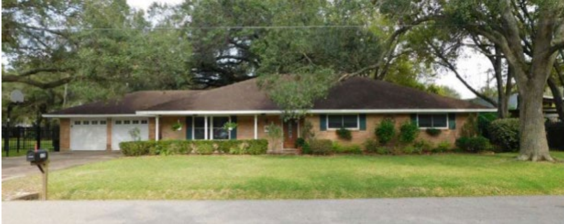
320 S. Kansas Avenue. This house is a typical one-story brick ranch house with an attached garage, low pitched roof with asphalt shingles, and wide eaves. There is minimal ornamentation other than the wooden porch supports and decorative shutters.
