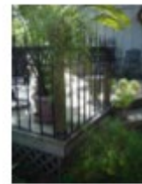
Wrought Iron w/ wood structural frame
