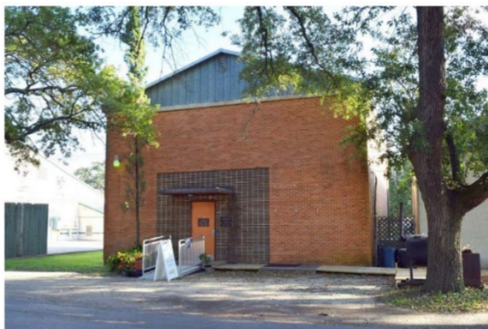
114 Park Avenue is an example of the Post-War Modern Style. Built in 1955, the building was previously used as the League City Masonic Lodge and is now used as a church.
