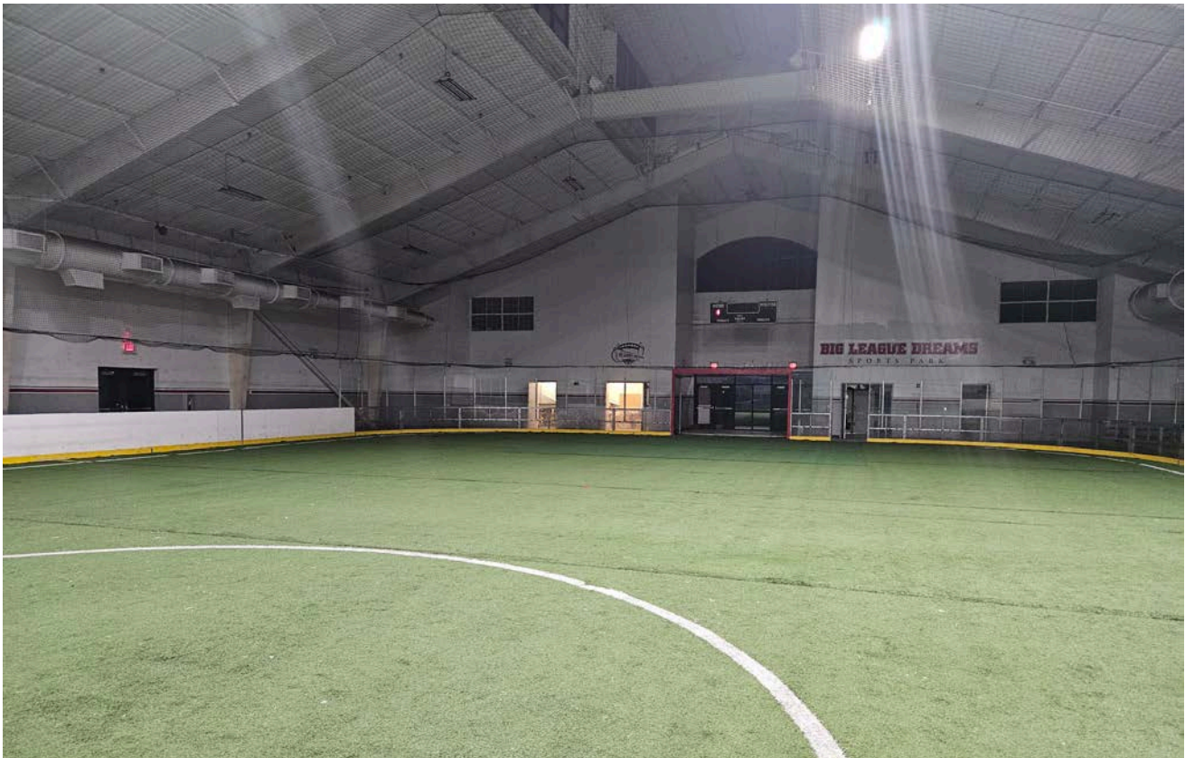
The images above illustrate the condition of the indoor turf field building at the time of KemperSports' facility assessment.
