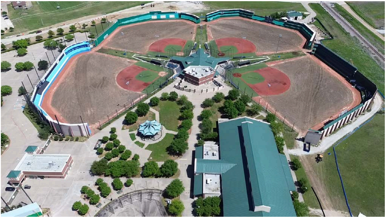
The images above show renovations underway, with fields prepared for geotechnical assessments to support full-field synthetic turf installation.
