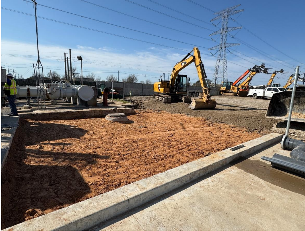
Manhole installation and backfill complete
