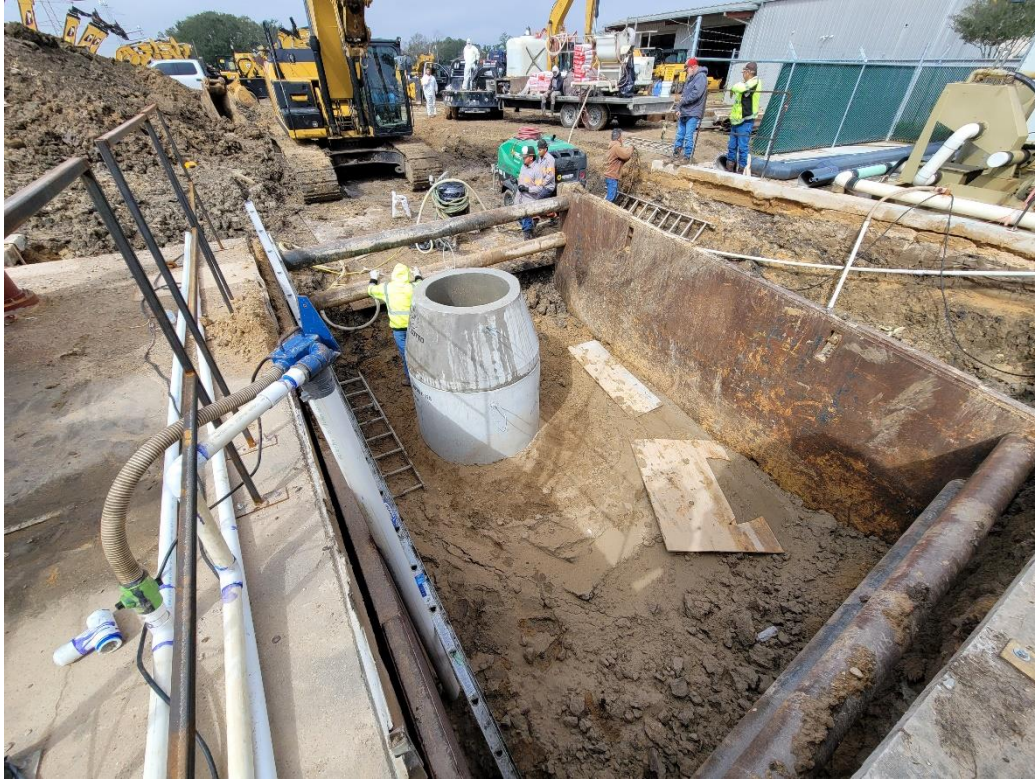
Backfill of manhole an installation of manhole cone
