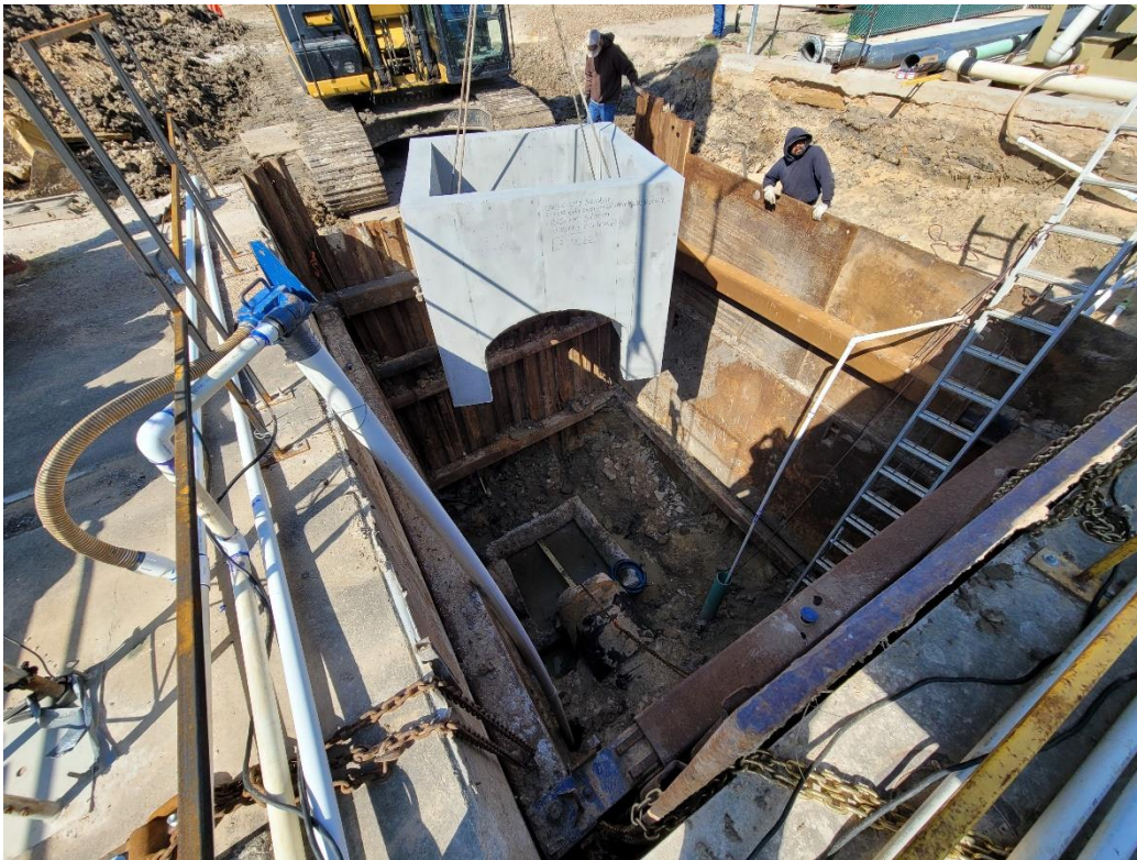
Installation of manhole base
