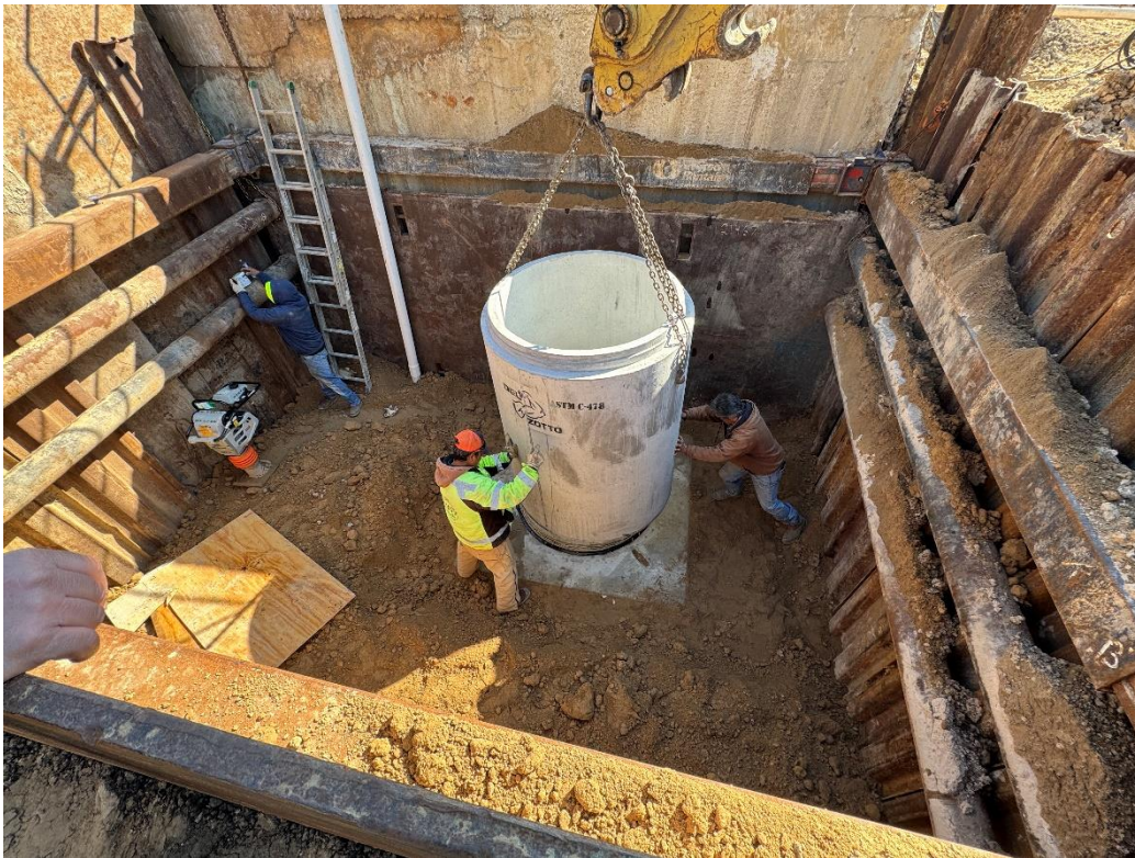
Installation of manhole cone
