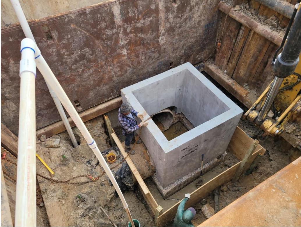
Manhole base installed
