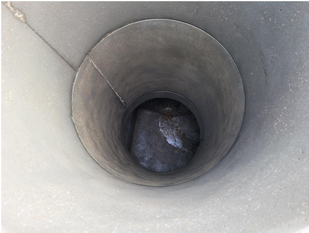
Installation of SewperCoat Lining
