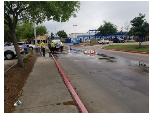
Overflowing sewer manhole behind FM646 restaurant strip.
