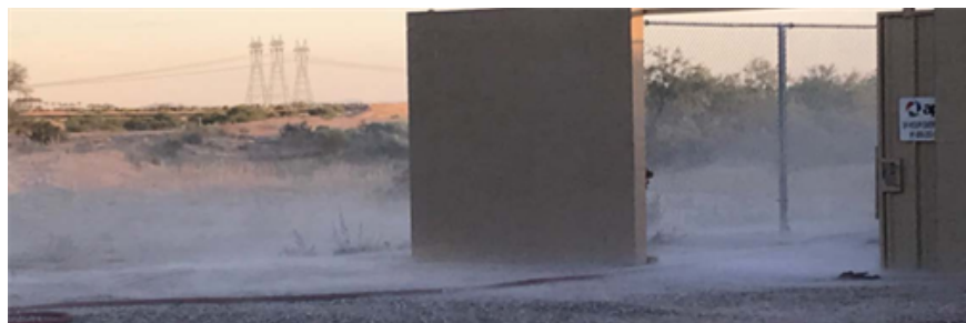
Figure 3: Smoke and gas at the APS McMicken site in Surprise, Arizona.
