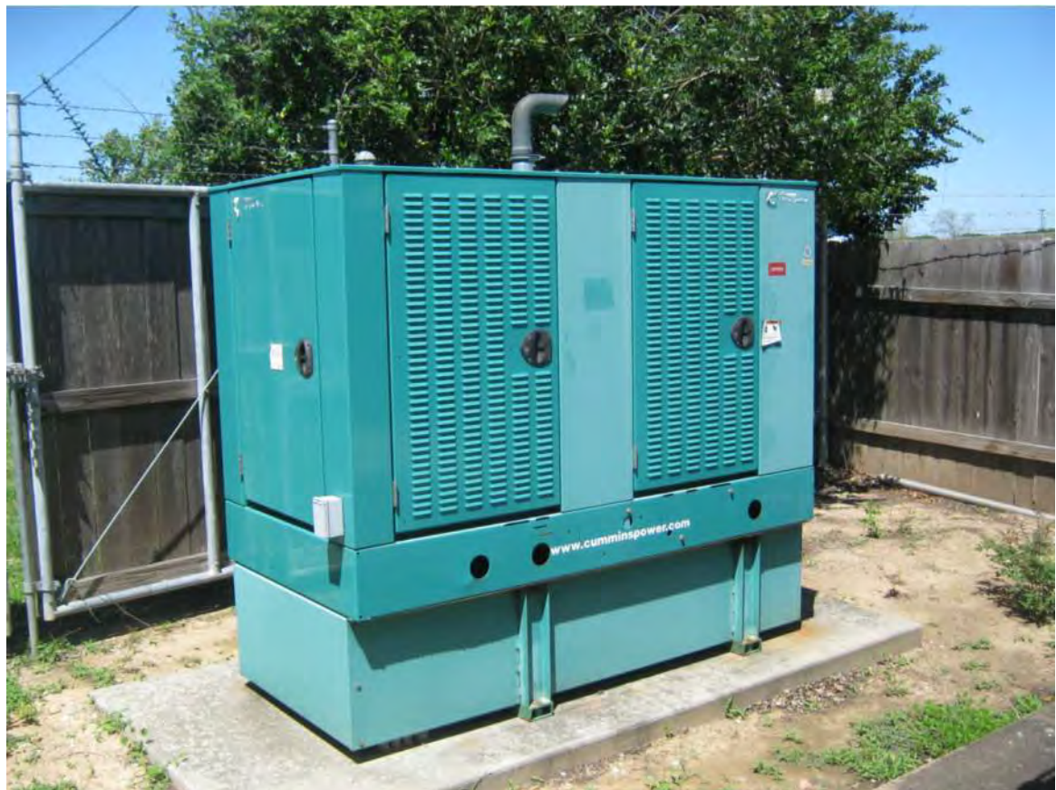
STAND-BY GENERATOR - DEMOLITION NOT TO SCALE
