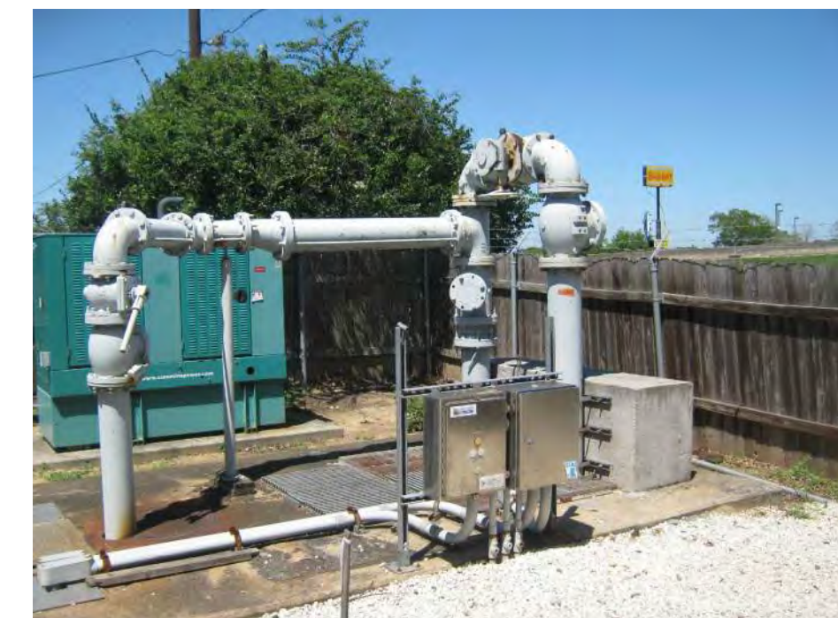
EXISTING LIFT STATION DISCHARGE PIPING
