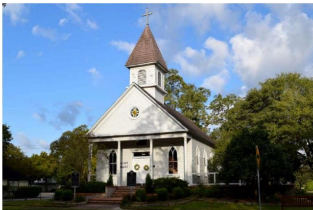
St. Mary Mission Church 620 E. Main Street Dedicated in 1920, this church is an intact example of the Carpenter Gothic style. Characteristics include frame construction, wood cladding, steeply pitched roof and pointed arch windows.
