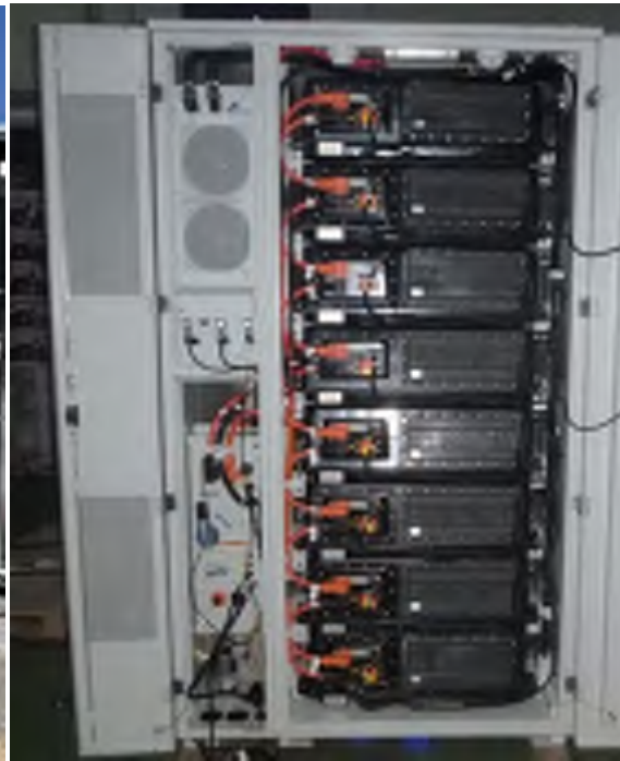
4.5ft x 4.5ft liquid-cooled enclosures
