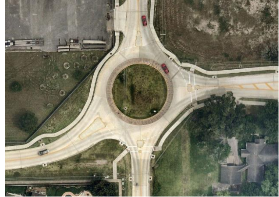
Figure 65: Existing Roundabout at Turner St and Butler St in League City
